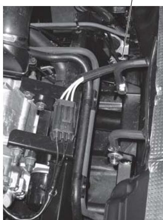
Power Fuse Box
